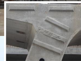
Use of segments with damaged shear keys is not a good practice.
