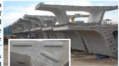
Use of segments with damaged shear keys is not a good practice.
